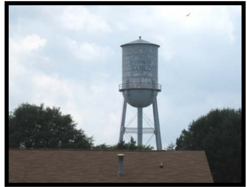
Elevated storage tank
